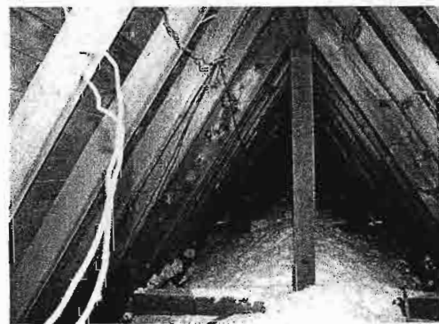
Figure 31. Kingston, St. Paul's Anglican; details of roof boards and supporting beams taken from inside the tower; Paul Christianson, 2010.
